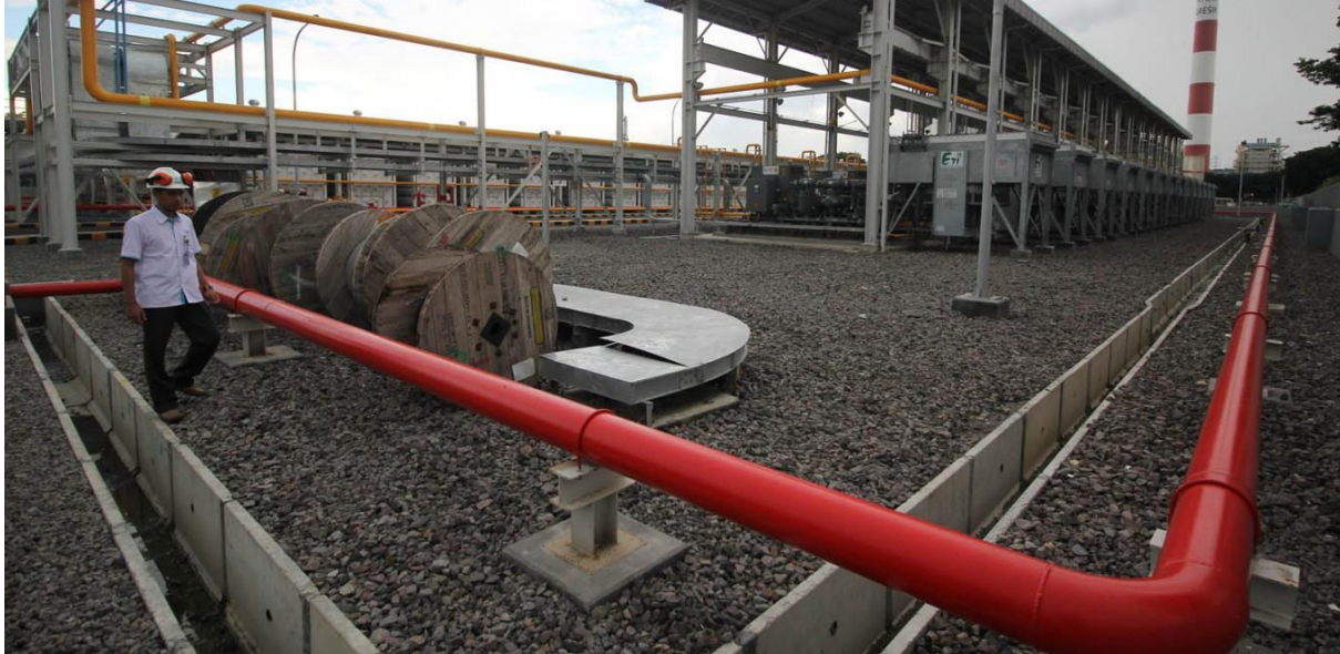
A worker inspects a gas pipeline. (Antara Foto/Moch Asim)
