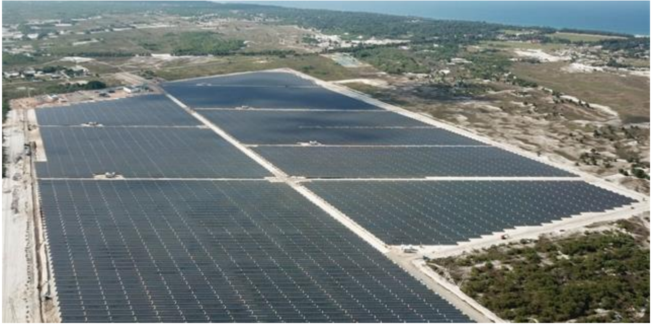
The LIG Solar Power Plant in the central province of Quảng Trị (Photo dientungaynay.vn)
