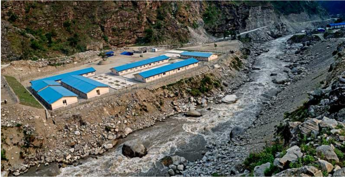
The campsite in Mailung, Rasuwagadhi, will house contractors and engineers during construction of UT-1, which will start by 2020.
