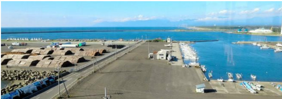
An offshore wind farm will be built near the outer seawall off Noshiro Port in Akita Prefecture (Yoichi Masuda)
