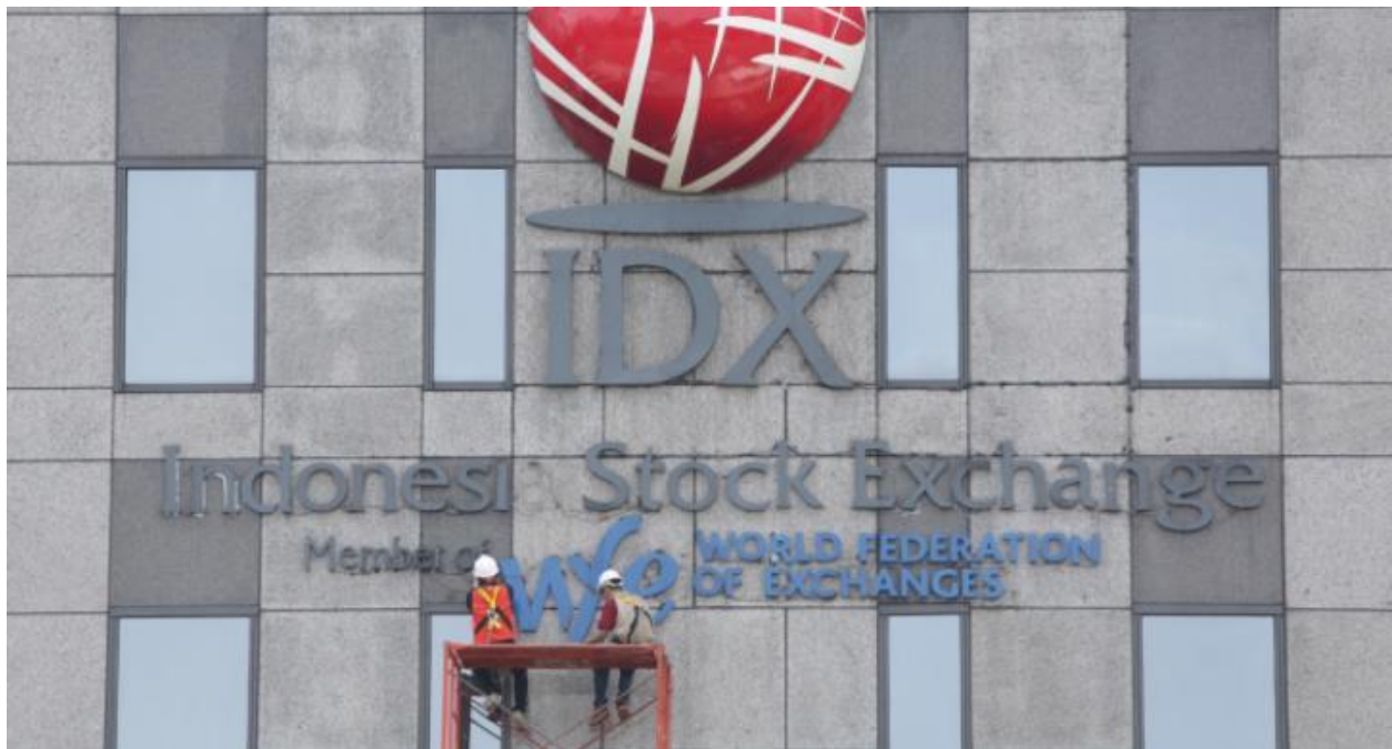
Workers maintain the Indonesia Stock Exchange (IDX) building in Jakarta
