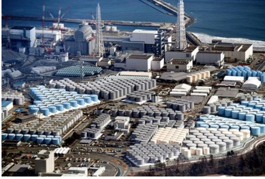
Hundreds of storage tanks on the grounds of the crippled Fukushima No. 1 nuclear power plant contain water contaminated with radioactive materials. (Asahi Shimbun file photo)
