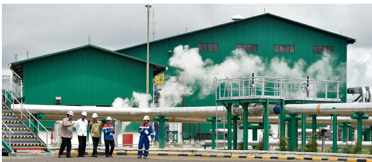
President Joko "Jokowi" Widodo (second left) visits a geothermal power plant in Tompasso, Minahasa regency in North Sulawesi. (Antara/Puspa Perwitasari)
