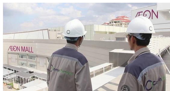
The huge Aeon Mall, situated in central Phnom Penh, is covered in solar panels
