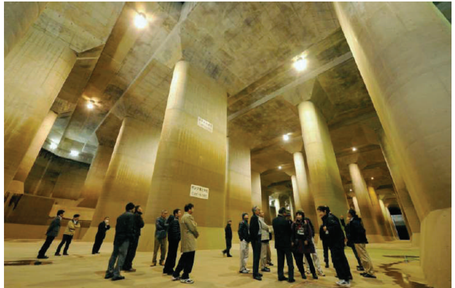
Visitors examine the Metropolitan Area Outer Underground Discharge Channel, in Kasukabe, Saitama Prefecture.
